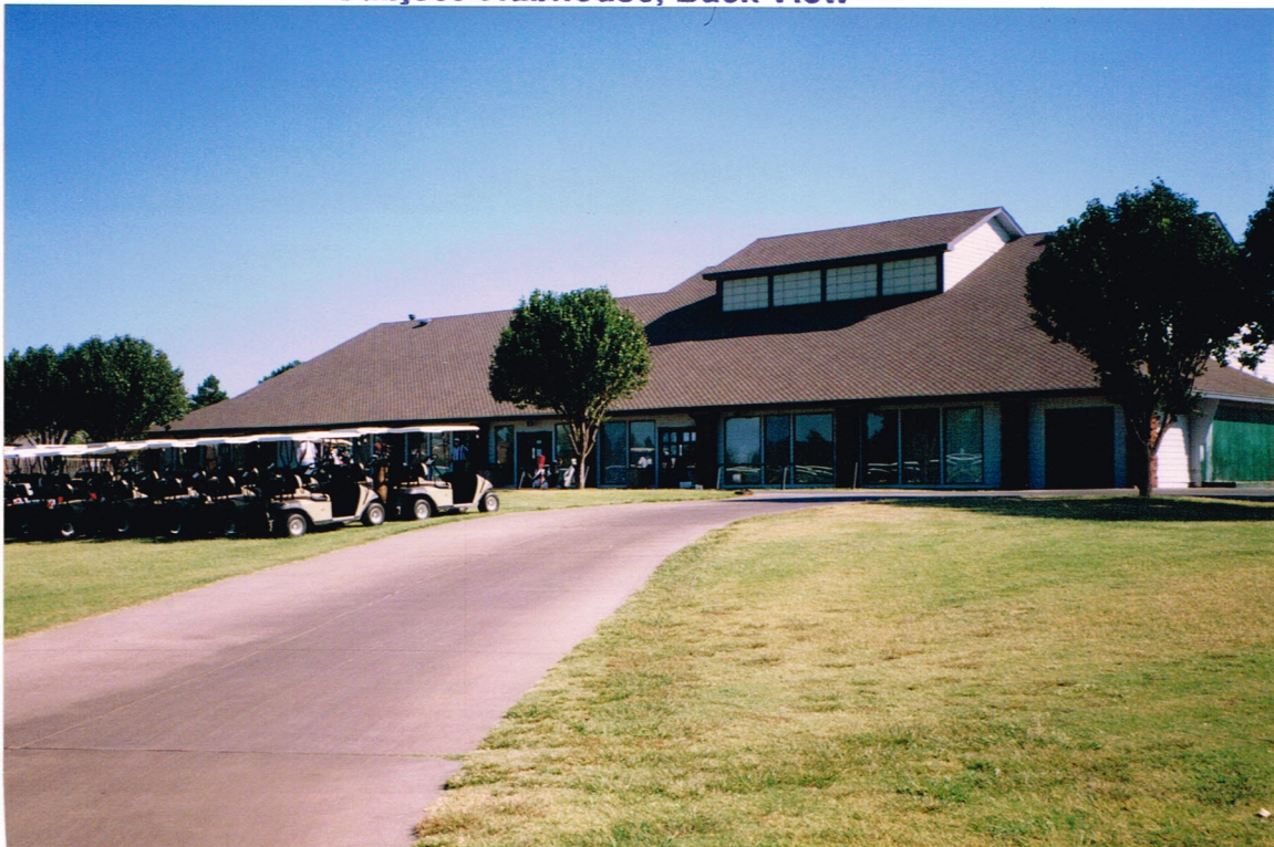
Subject Clubhouse, Back View
